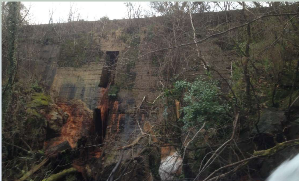
← The wall of the tailing dam nº 2 is 50x12,5 m (length x high).
